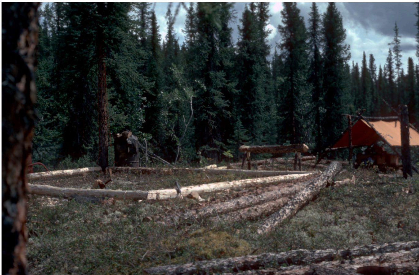
Setting the foundation logs for Broken Skull cabin.
