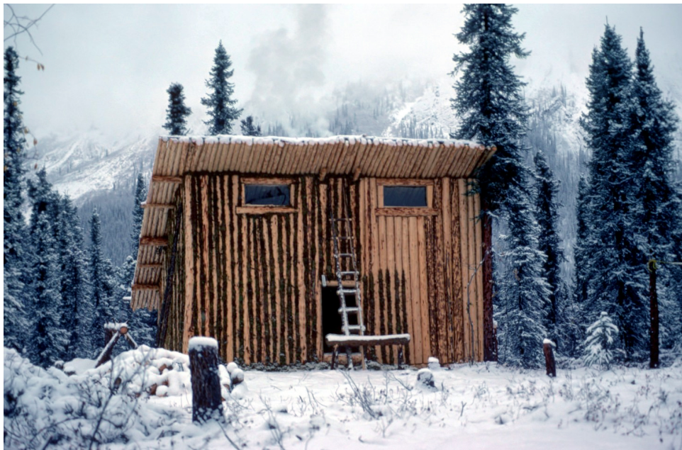
Moss chinking being applied to the south wall.
