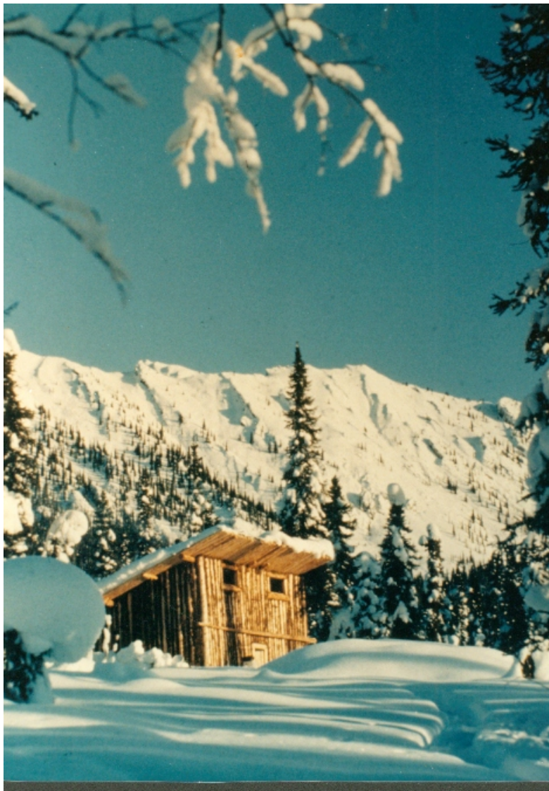
The completed cabin at Broken Skull.
