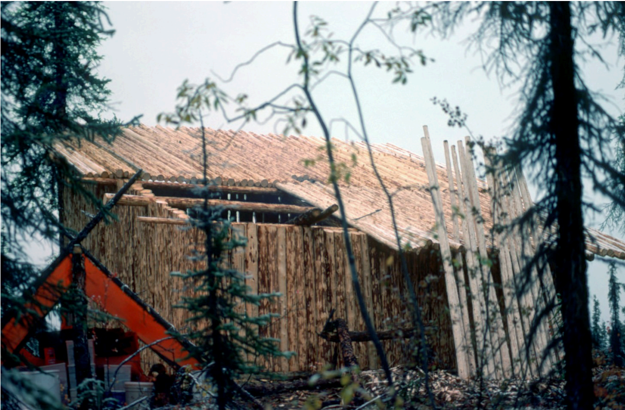
Cabin roof construction.
